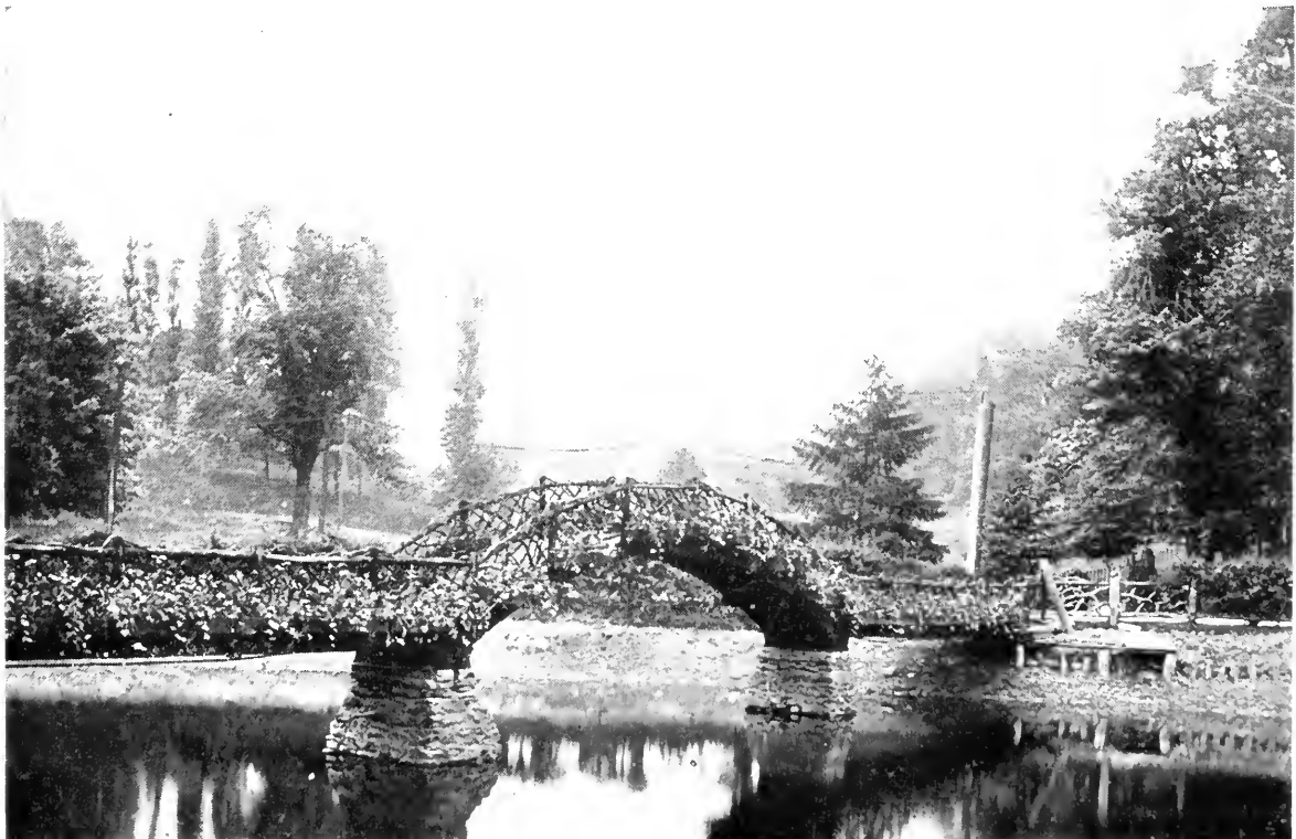
A light rustic bridge resting on substantial stone piers. The floral decoration is in full bloom.
